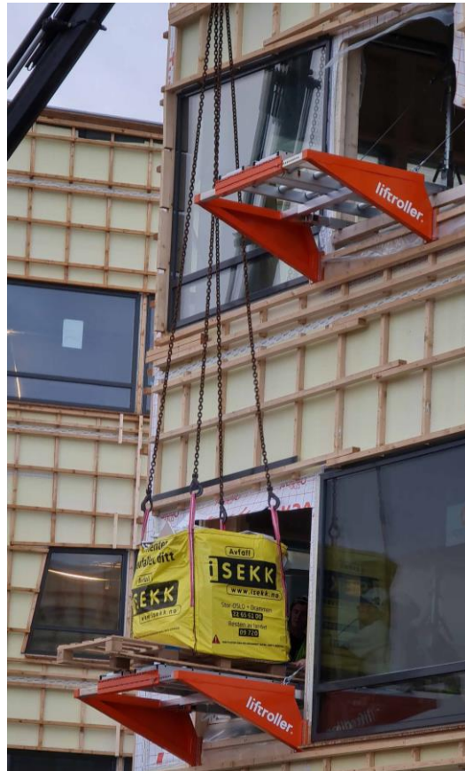
Kilen Office Building - Veidekke AS
