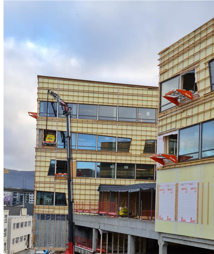
Kilen Office Building, - Veidekke AS
