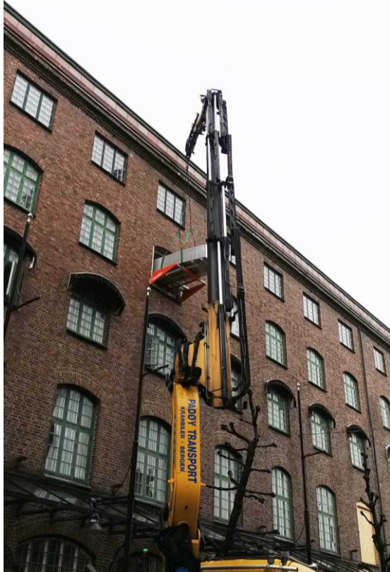
Abora Prosjekt AS - Office Building, Bergen
