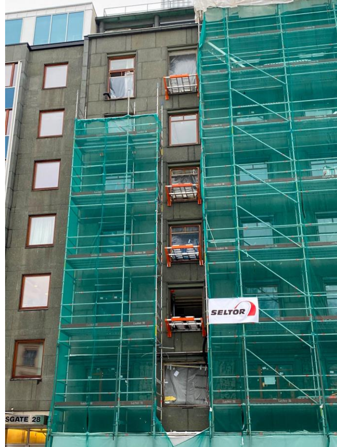
Seltor AS – Office Building KA 23
