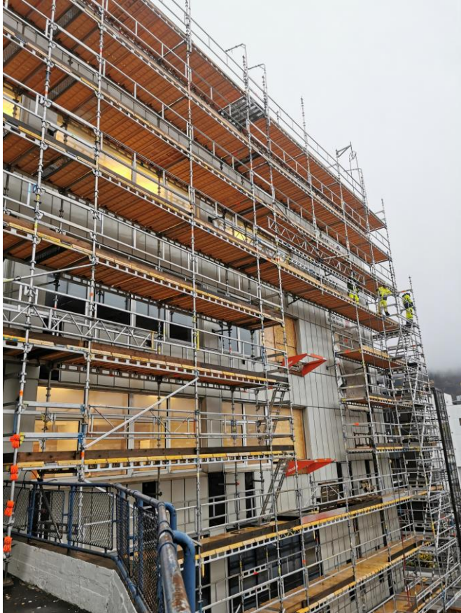
OBAS AS – Office Building, Bergen
