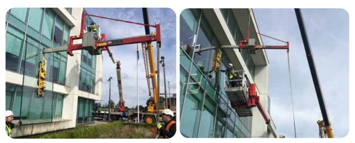
\*use of below-the-hook vacuum lifters depend on type of project. Below the hook lifter not included.
