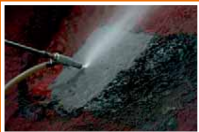
Surface - Sand Blasting
